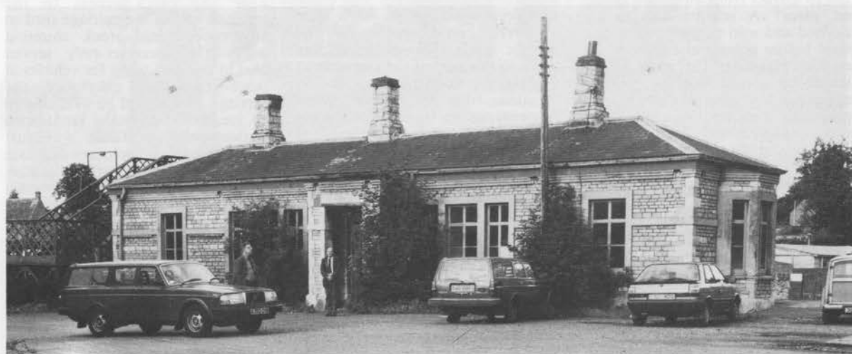
A visit to Heyford after the Society AGM on 14th July 1984. This building was dismantled by Society members in 1985/6. Careful siting and screening will ensure that when rebuilt, complete with restored all-round canopy, it does not overpower the northern part of the Didcot site.
