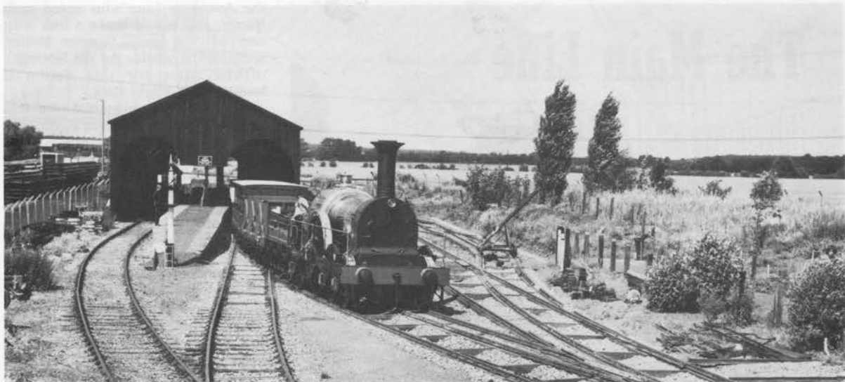
The space on the right, between the broad gauge and the site fence, has to accommodate a forecourt, station building, Main Line platform and the track itself—just possible by careful attention to layout and levels.
